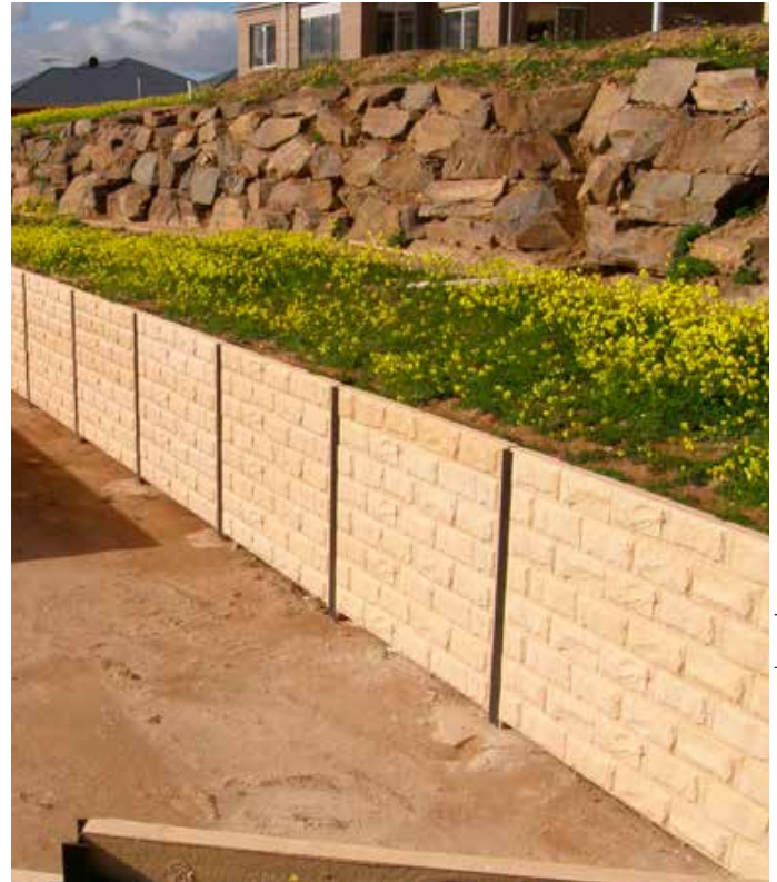
Concrete Sleepers | Bedrock Sandstone
